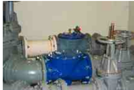
Now a Val-Matic Swing-Flex is working on both lines.
