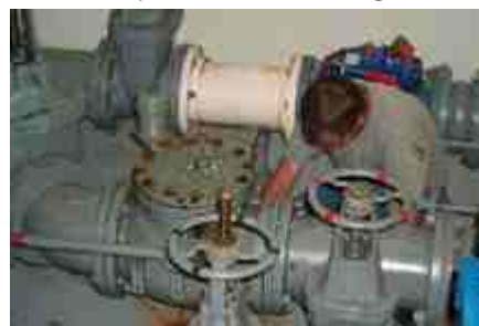
The old valve is removed.
