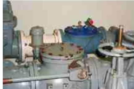
The Val-Matic Swing-Flex Check Valve was already used once to replace the "other" valve. Operators liked it so much they ordered another.
