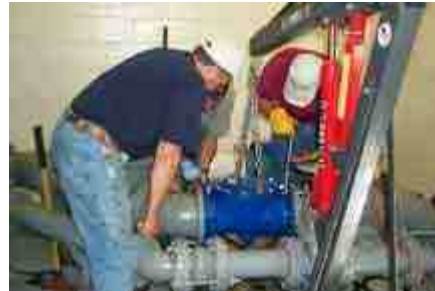
The new Val-Matic Swing-Flex is installed.
