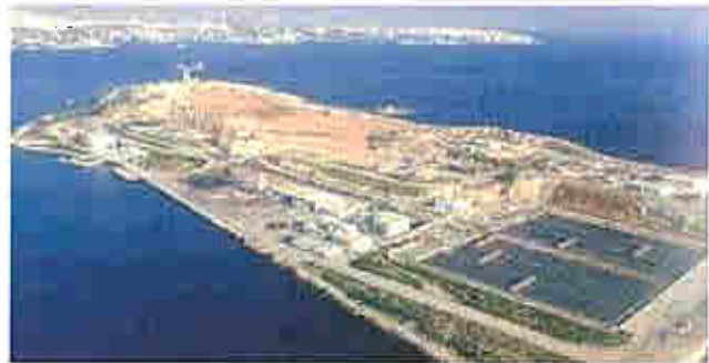
Psyttalia Wastewater Treatment Plant
